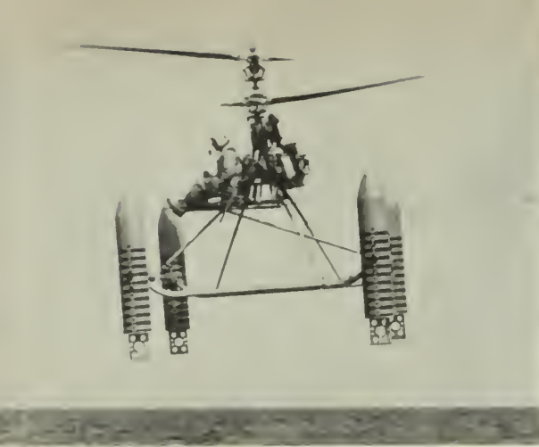
ROUGH CUSTOMER —Photo series shows floats positioned for land operation and flight, and for rough water landing.
